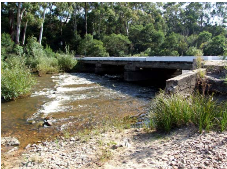
The Oallen Ford bridge on the Shoalhaven River
