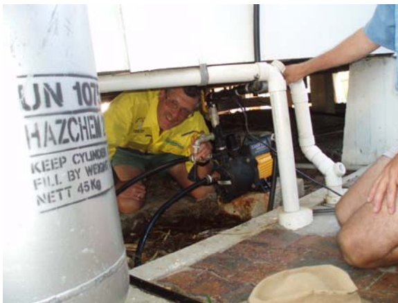
The Master’s Apprentice – Installing a water pump with Ian
